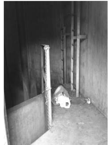
ladders inside the storm drain area
