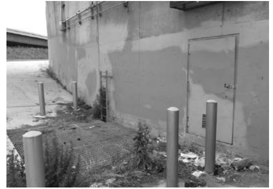
the access door to the storm drain area
